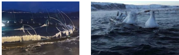
Fig. 1. Damage to fish farm cages caused by ice accretion in Northern Norway (Picture: Alexander Boiko).
